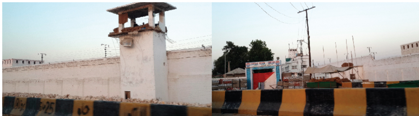
(Picture of the boundary wall of Central Prison, Sukkur) 91 .
