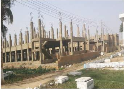
New Double Storey Barracks under Construction at District Prison, Malir 64
