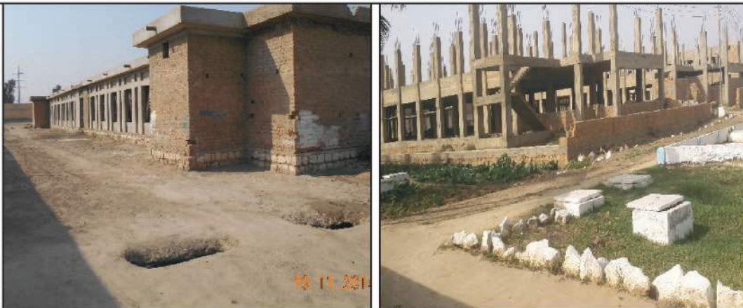
New Barracks Being Constructed In Larkana District Prison 63
