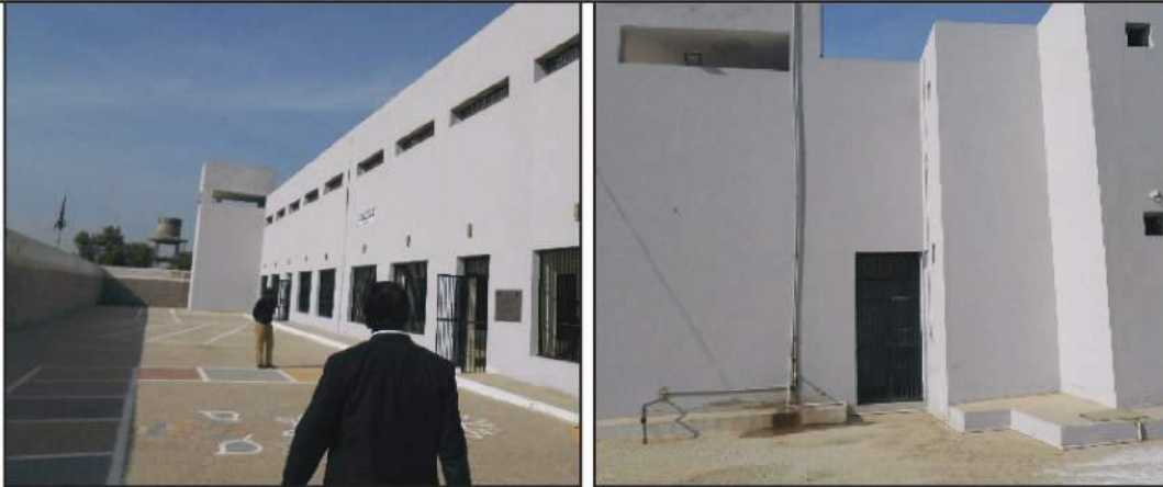
New Double Storey Barracks Constructed in Khairpur Central Prison 62
